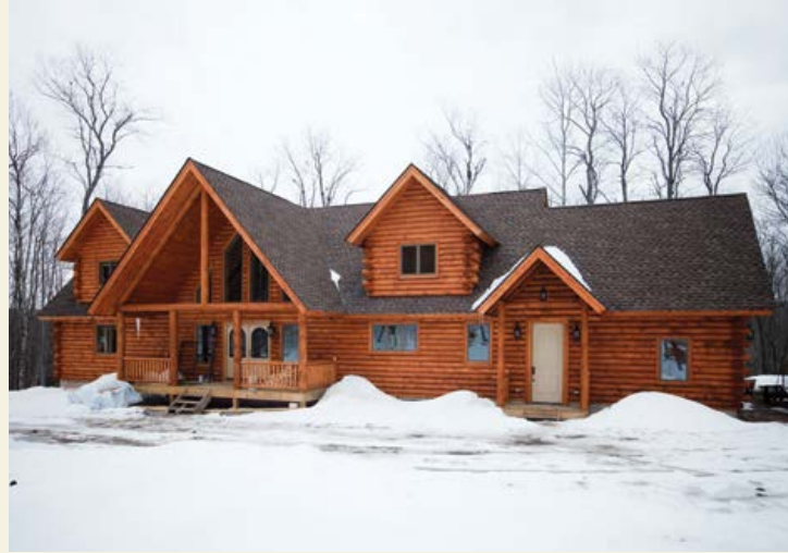
One of the homes currently under construction on Tanzman Lake
