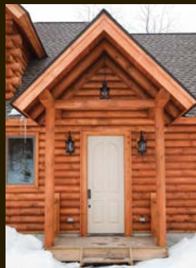
Detail of a porch with timbers
