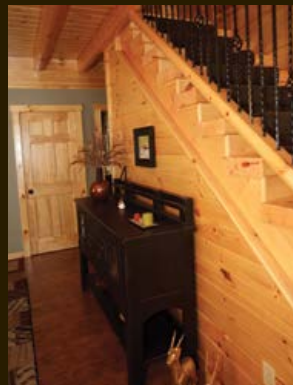
Detail of a custom wrought iron stair railings
